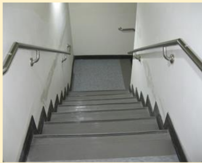
Accessible stair handrail
