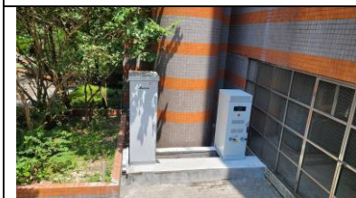
Figure 6: Setting up a battery storage system to maximize the benefits of electricity usage
