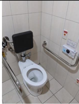
Accessible facilities in dormitory toilets
