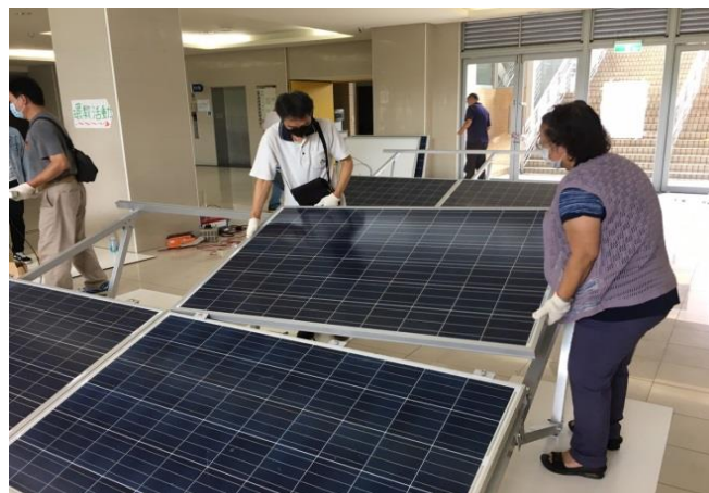
Caption: Assembling solar panels
