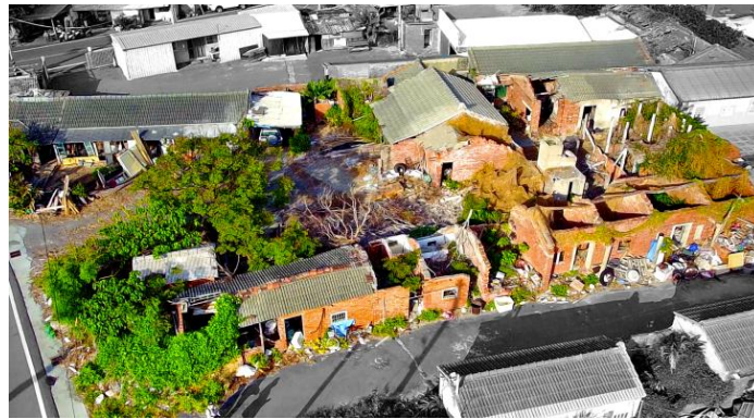
Figure 8. Aerial photograph of abandoned sanheyuan (traditional courtyard houses) in the Fangyuan area of Changhua County.
