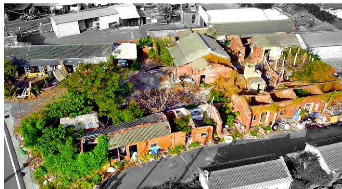
Figure 2. Aerial photograph of abandoned sanheyuan (traditional courtyard houses) in the Fangyuan area of Changhua County.
