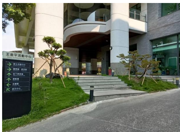
Figure 1. The yew plum pine and Chinese juniper planted next to the staircase leading to Wang Jin-Ping Activity Center
