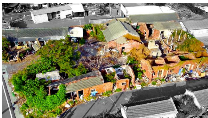
Figure 4. An aerial photo of abandoned sanheyuan (traditional courtyard houses) in Fangyuan, Changhua County
