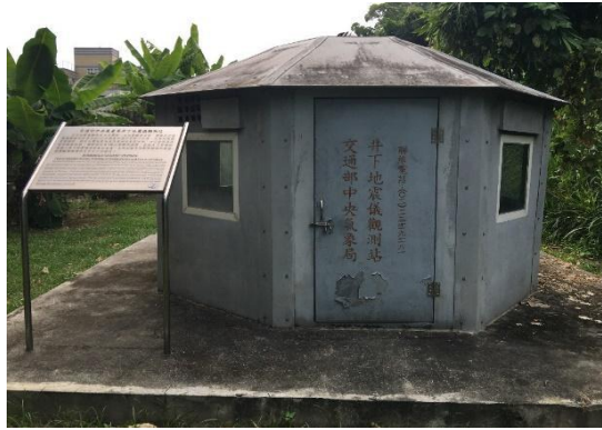
Figure 11. Underground seismograph observation station in residential areas. The seismograph installed at a depth of 300 meters in the well can significantly reduce the interference from surface noise and obtain high quality ground motion signals, improving the accuracy of seismic locating and the ability to monitor regional small-scale earthquakes
