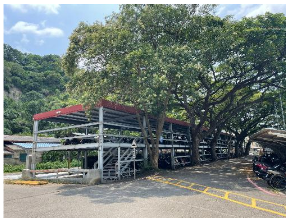
Figure 1. Multi-Story Motorcycle Parking Tower at the West Side Entrance of NCUE
