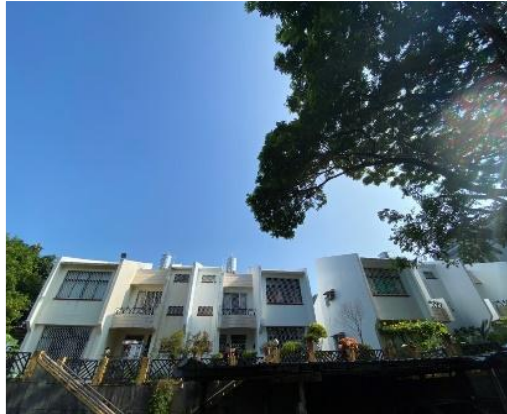
Figure 2. Dormitory Building Exterior
