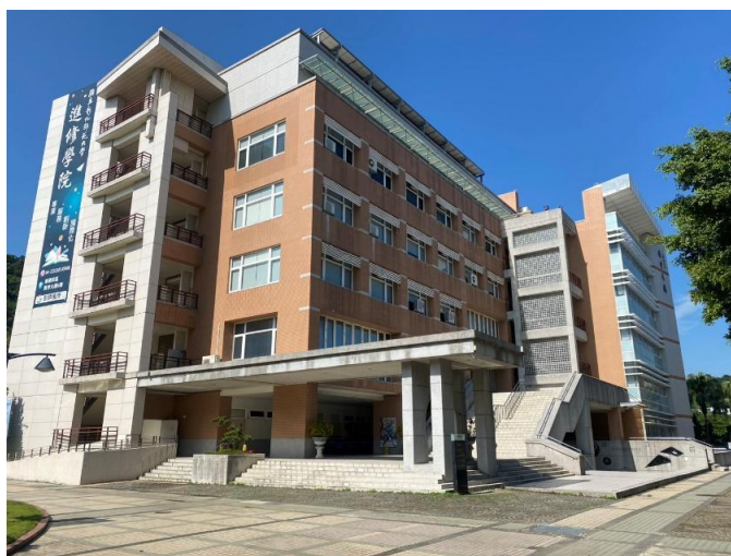
Figure 2. NCUE Teaching Building, Jinde Campus
