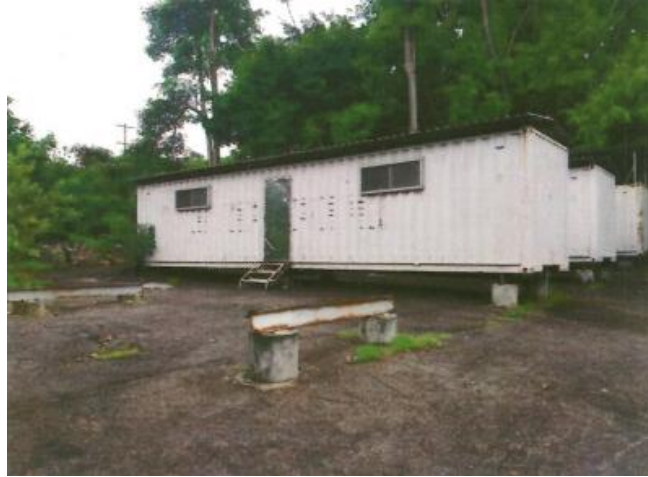
Figure 2. Former Unused Container Houses
