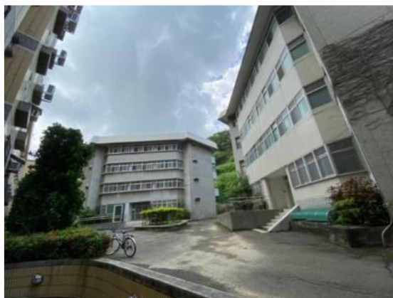
Figure 1. Dormitory Building Exterior
