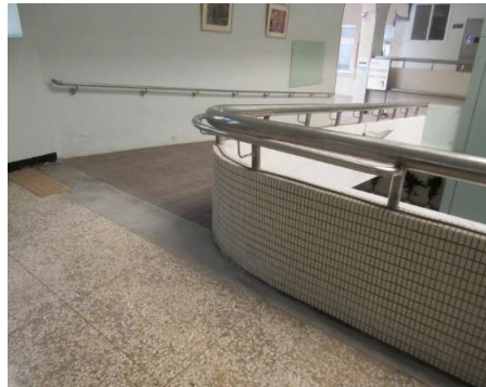
Figure 9: Handrails for accessible ramp
