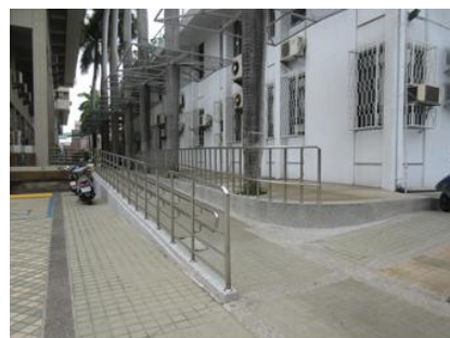
Figure 6: Accessible ramp with service bell
