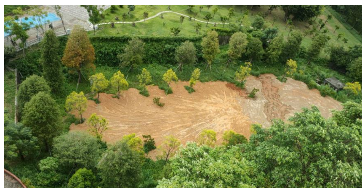
Figure 12: Detention basin at the Baoshan Campus
