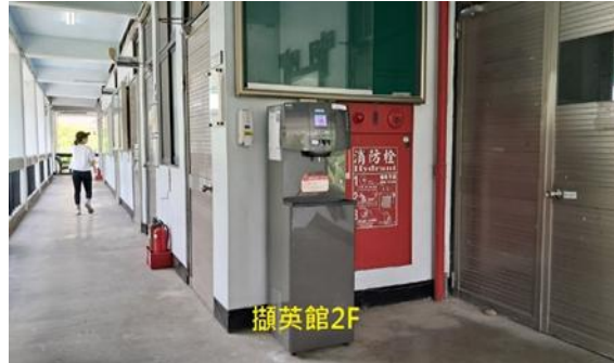
Figure 1. Water dispenser on the 2nd floor of the Jieying Building on the Jinde Campus
