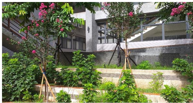
Figure 7. Baoshan Campus - Sprinkler irrigation system is in the flower bed of Student Dormitory No. 10
