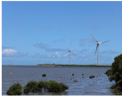
Figure 11. Wind Turbines along Fangyuan Coast
