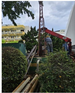
Figure 2. Workers were repairing the deep water well at Jinde Campus
