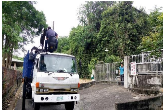
Figure 13. Sludge removal operations on Baoshan Campus's sewage treatment plant
