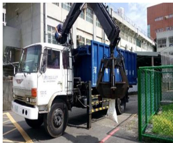
Figure 10. Sludge removal operations on Jinde Campus's sewage treatment plant
