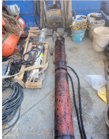
Figure 4. A deep water well motor to be repaired
