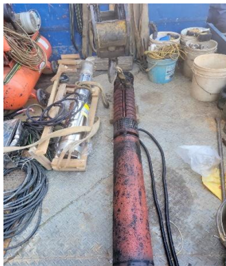
Figure 3. A deep water well motor to be repaired
