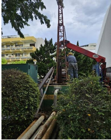
Figure 3. Workers were repairing the deep water well at Jinde Campus
