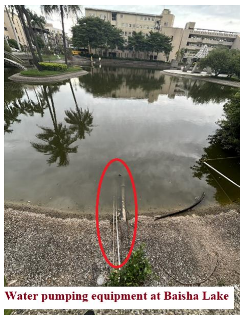
Figure 2. - Water Pumping Equipment at Baisha Lake
