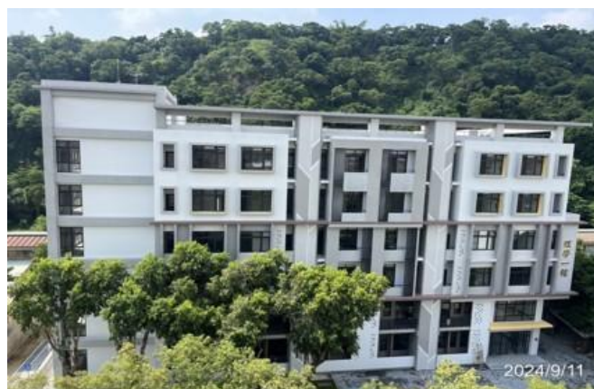
Figure 10. The first phase of the Building of College of Science construction project
