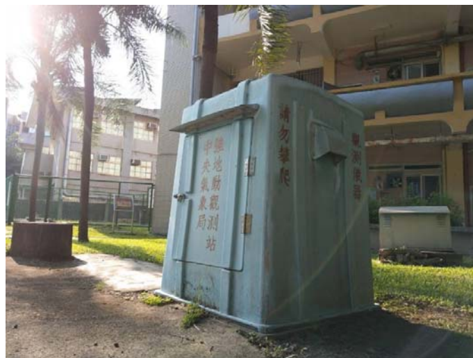
Figure 3. Strong motion observation station in Jinde Campus The observation station houses
