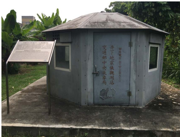
Figure 5. Underground seismograph observation station in family quarters. The seismograph installed at a depth of 300 meters in the well can significantly reduce the interference from surface noise and obtain high quality ground motion signals, improving the accuracy of seismic locating and the ability to monitor regional small-scale earthquakes
