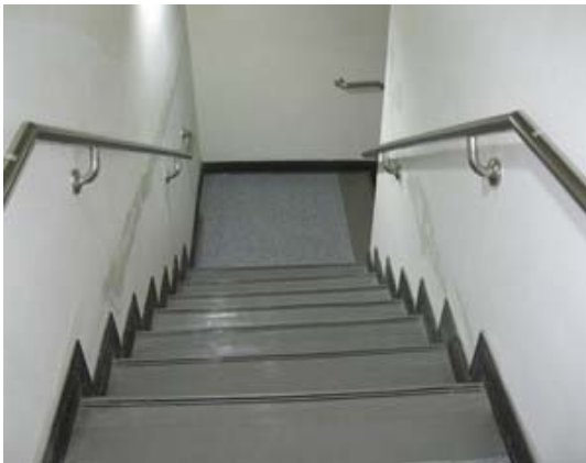
Figure 3. Accessible stair handrail
