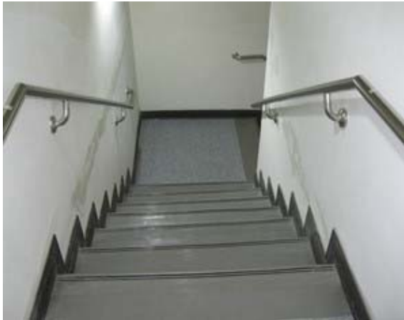
Figure 2. Accessible stair handrail
